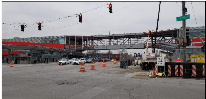
95th Street Terminal construction
