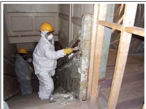
Lead being removed from a residential building.
