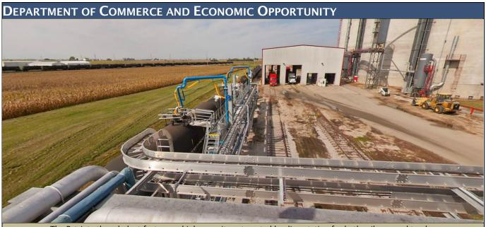
The Patriot ethanol plant features a high-capacity automated loading station for both rail cars and trucks.
